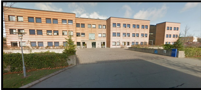
Figure 2 – Data center building entrance.
