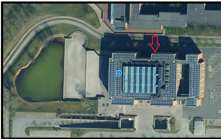
Figure 1 – Data center building in Aalborg.
