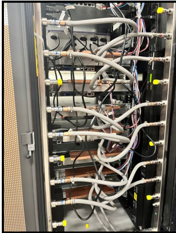
Figure 8 – Connection of HEATFLOW heat exchangers to the manifold.
